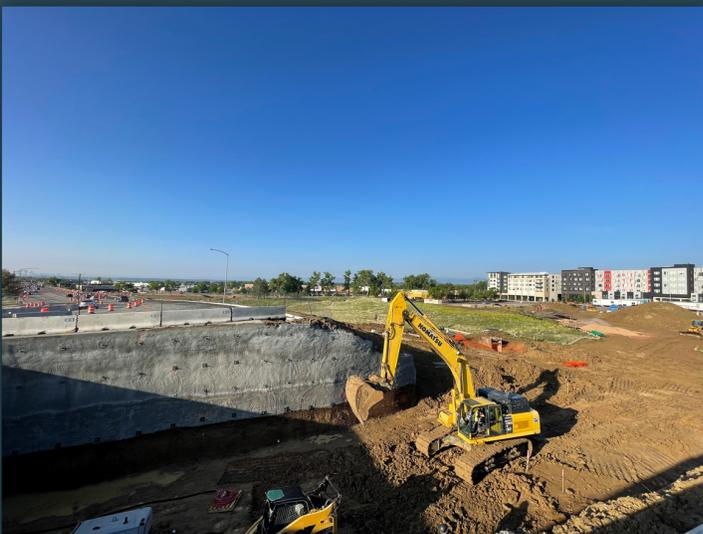
The Sheridan Boulevard Multimodal Transportation Improvement project is constructing a concrete pre-cast arch underpass beneath Sheridan at W. 89th Ave. which will connect Downtown Westminster to RTD's U.S. 36 & Sheridan Station and expand Sheridan to a six-lane road from Turnpike Drive to W. 88th Place. This \$9.3M project, \$6.6M of which is from Federal Funds, is planned to be completed in the Spring of 2023.
