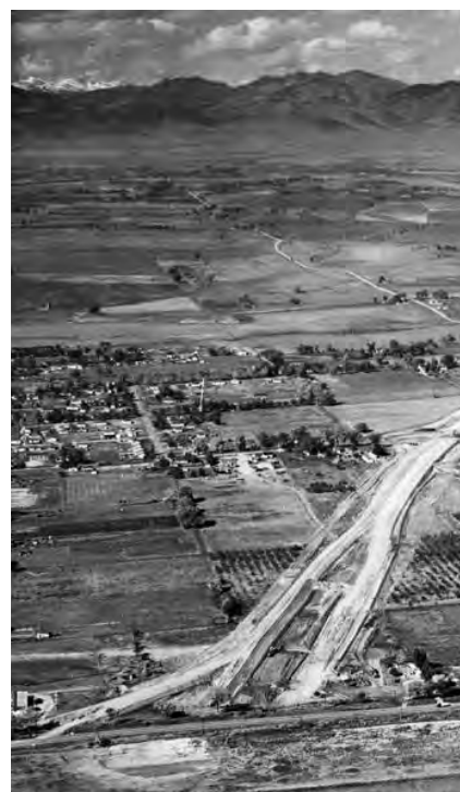
Turnpike Construction Photo credit: Carnegie Library for Local History in Boulder
