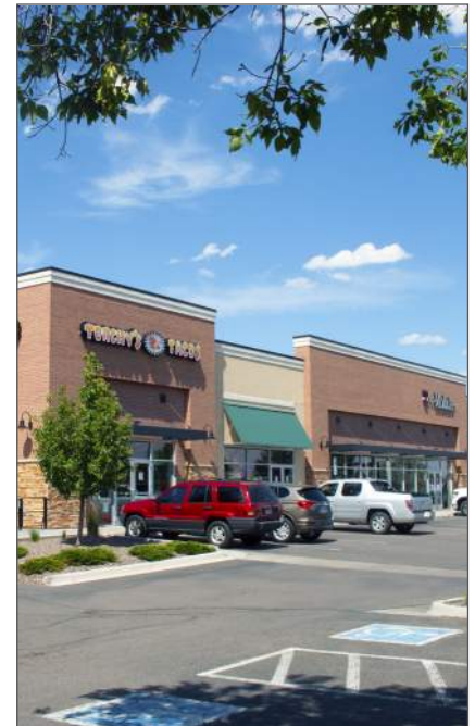
Towne Center at Brookhill
