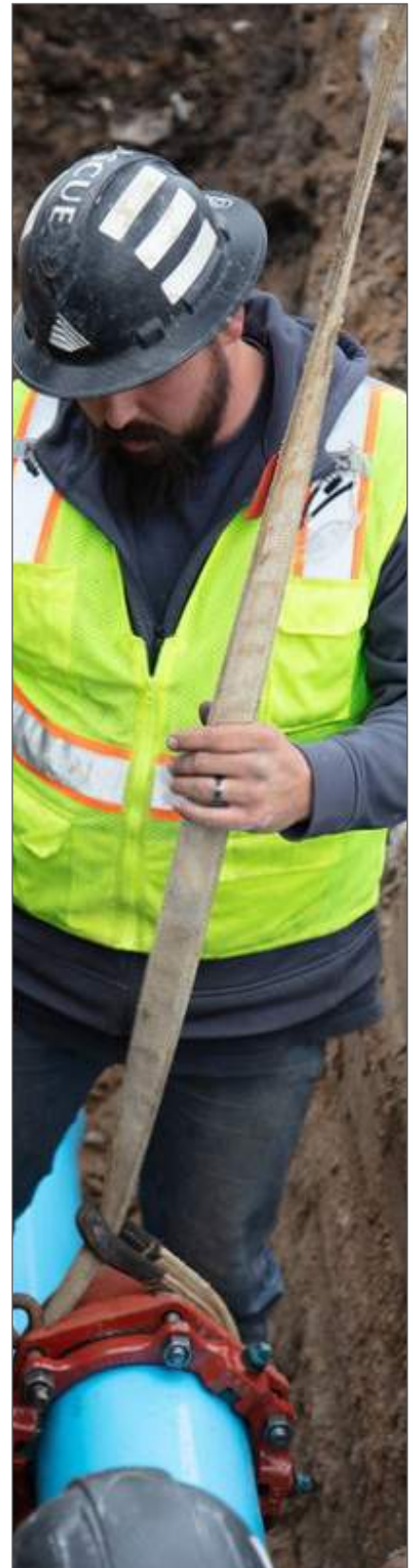
Water Main Replacement
