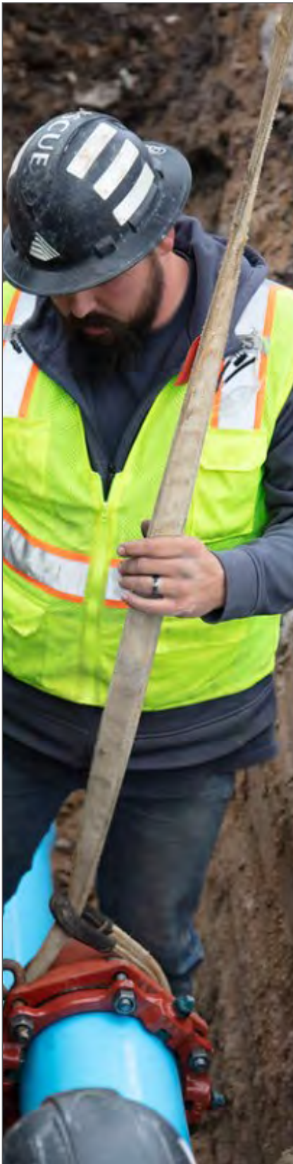
Water Main Replacement
