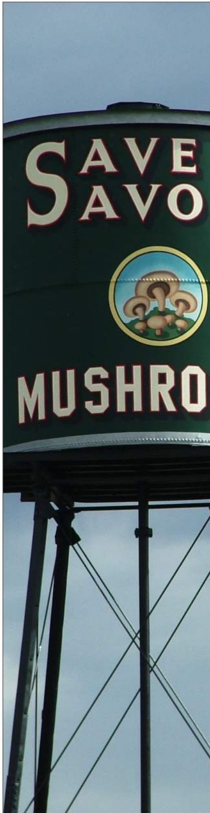
Restored Savery Savory Mushroom Water Tank
