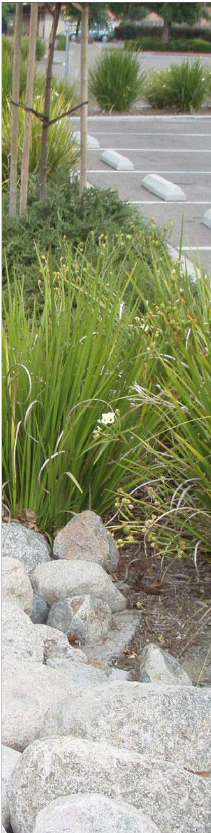
Parking Lot Bioswale
