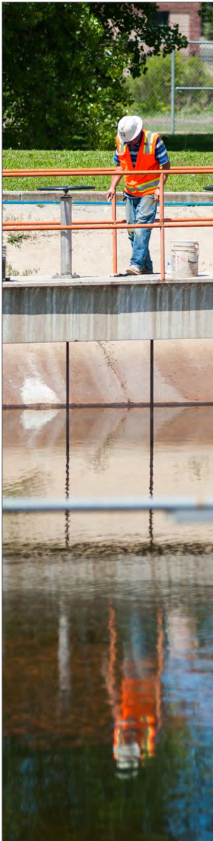
Semper Water Treatment Plant
