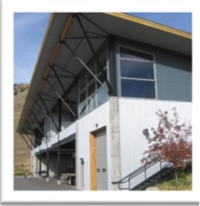
Small-Scale Industrial Warehouse
