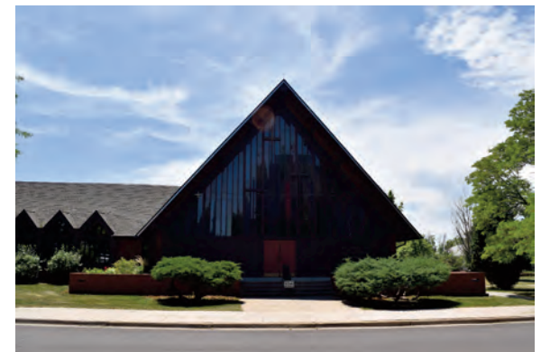
Figure 1.7. The 1957 Westminster Presbyterian Church exhibits many of the architectural characteristics of postwar churches. The geometric stained glass window defines the soaring gable face. The church also features some of the same materials, such as the stylized metal signage and the board-and-batten siding, used in construction of nearby Ranch homes. Not visible in the photo, there is a large parking lot (equivalent of over five house lots) to the east and a long, low, rectangular, International-style educational wing extending from the southeast corner of the church building. (Mary Therese Anstey)
