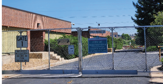
Aging Semper Water Treatment Facility, Built in 1969
