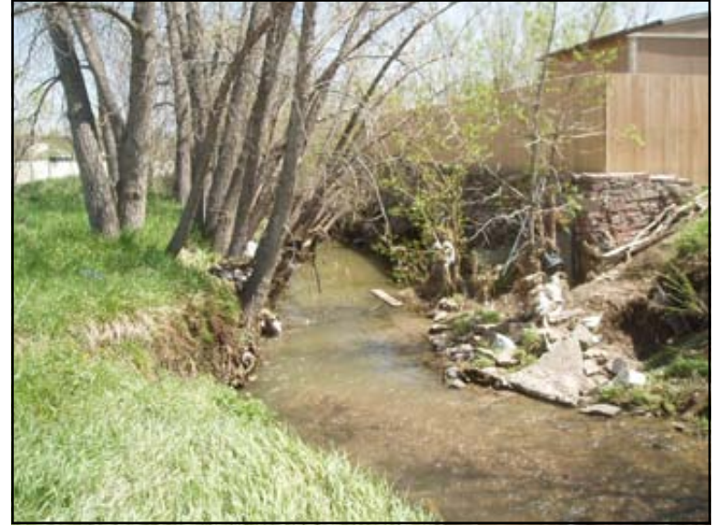
P4270019—Private Property on Edge of LDC w/ Bank Protection
