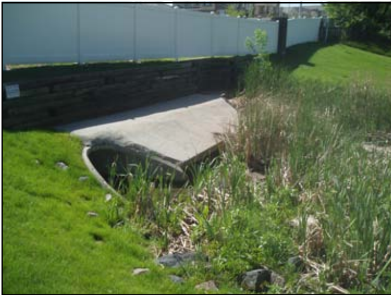
P5240007—Pecos St. Crossing Outfall
