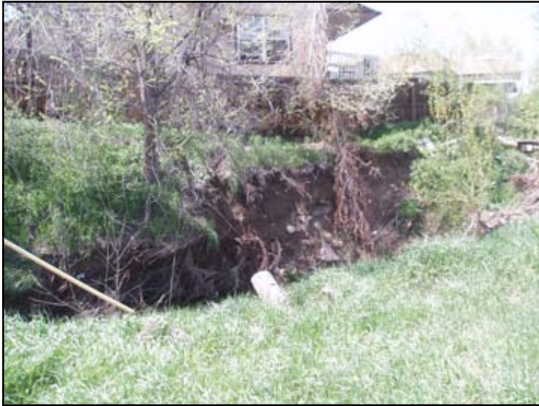
P4270018—House Close to 15' Bank Cut
