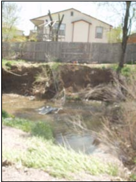
P4270020—House close to 15' Bank Cut
